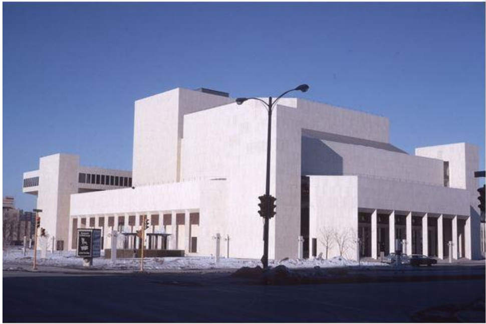
MARCUS CENTER BEFORE REMODELING
