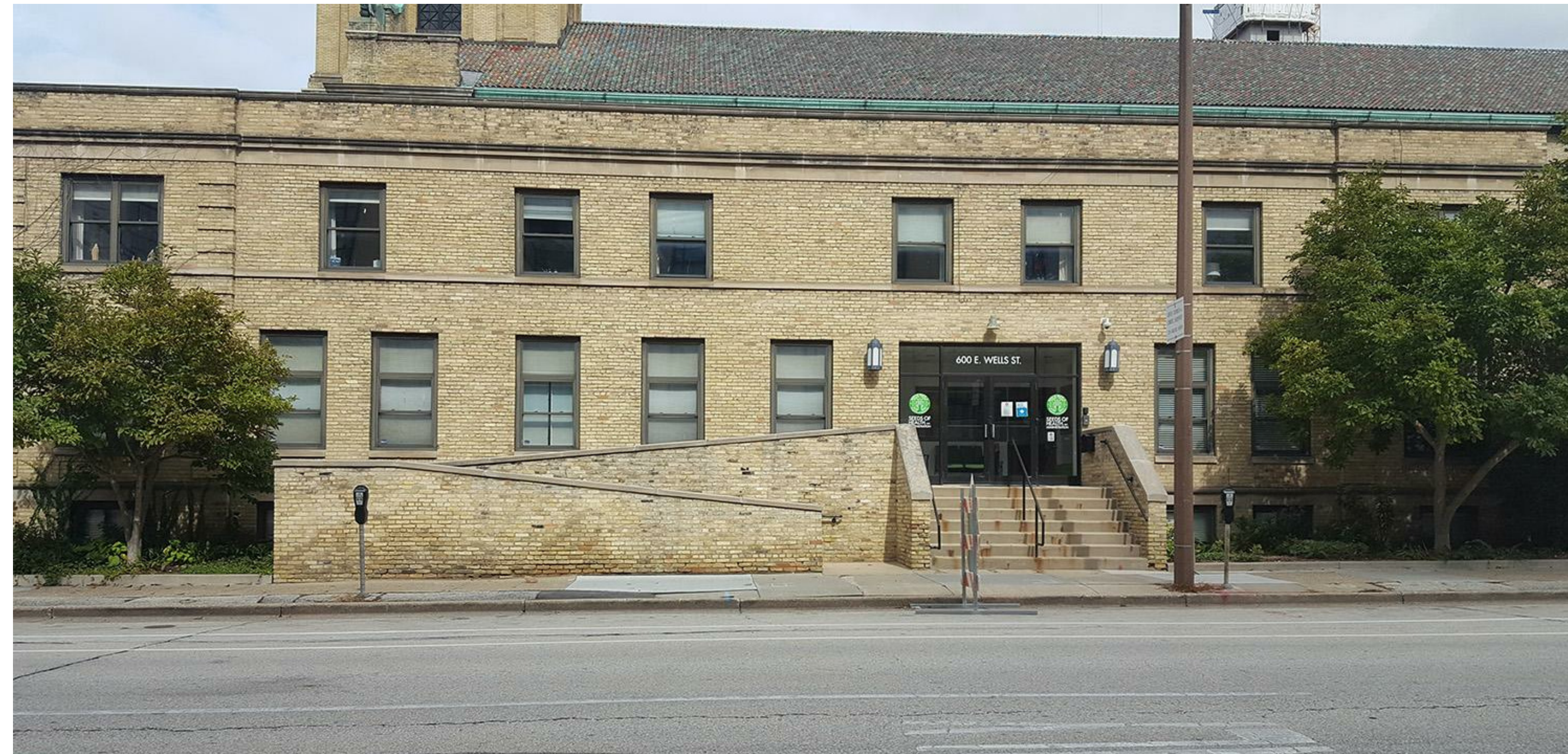
EXISTING PHOTO OF EAST ELEVATION.
