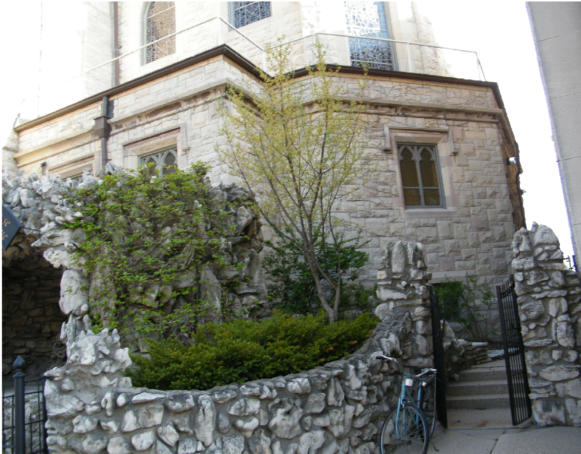
EXISTING SACRISTY ARCHITECTURE
