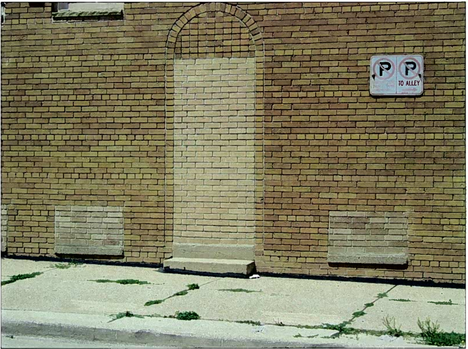
2972-74 South 13th Street CCF 080297 8/1/08 Looking North on West Manitoba Street at the concrete step
