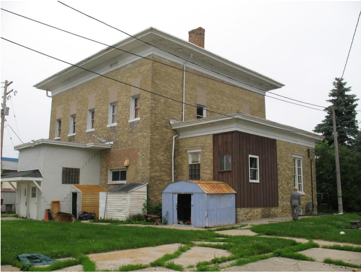
Jacob Nunnemacher Estate / Wildenberg Hotel Rear Elevation Looking Southwest
