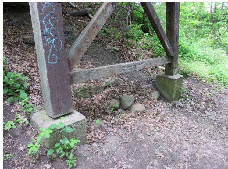
Photo F. Wood Columns/Concrete Piers.
