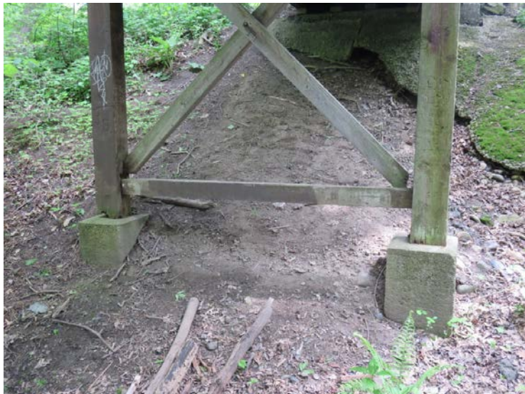
Photo E. Wood Columns/Concrete Piers.
