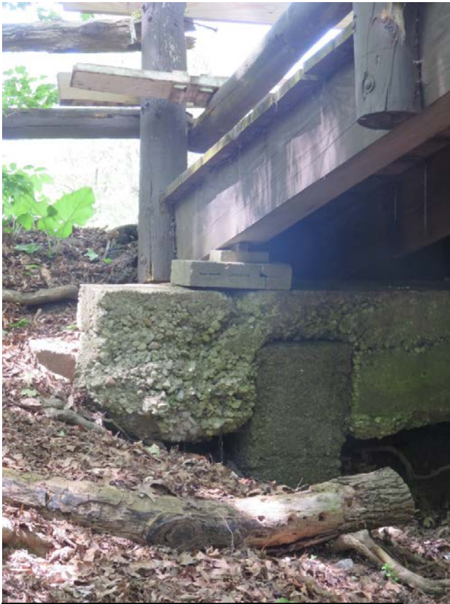
Photo C. North Concrete Foundation.
