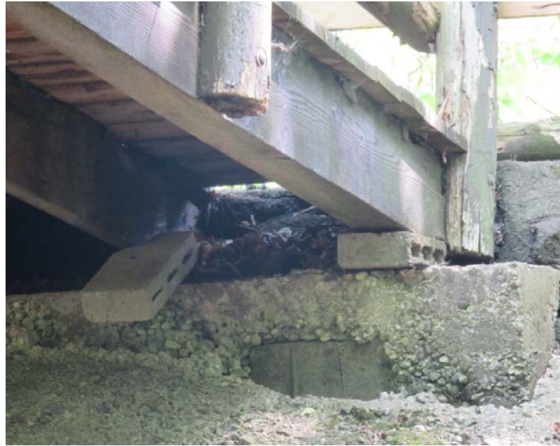
Photo D. South Concrete Foundation.
