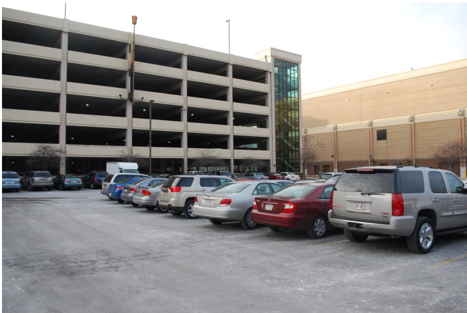
North West View from Parking Structure Site
