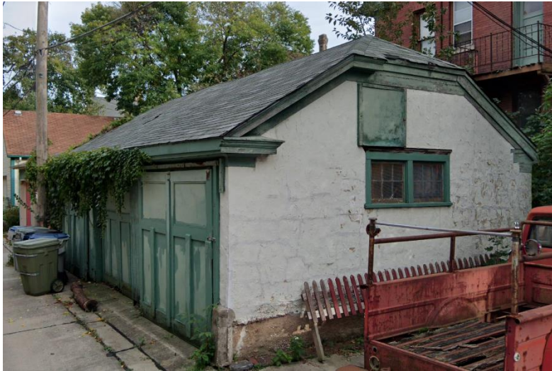
Existing garage roof
