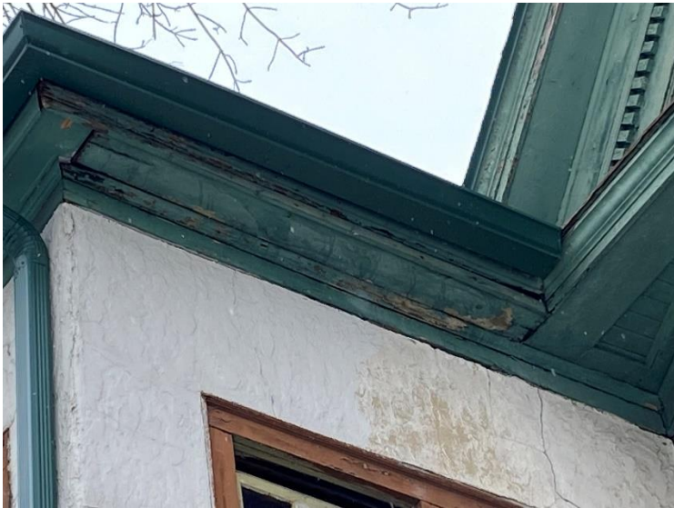
Existing damage to soffit
