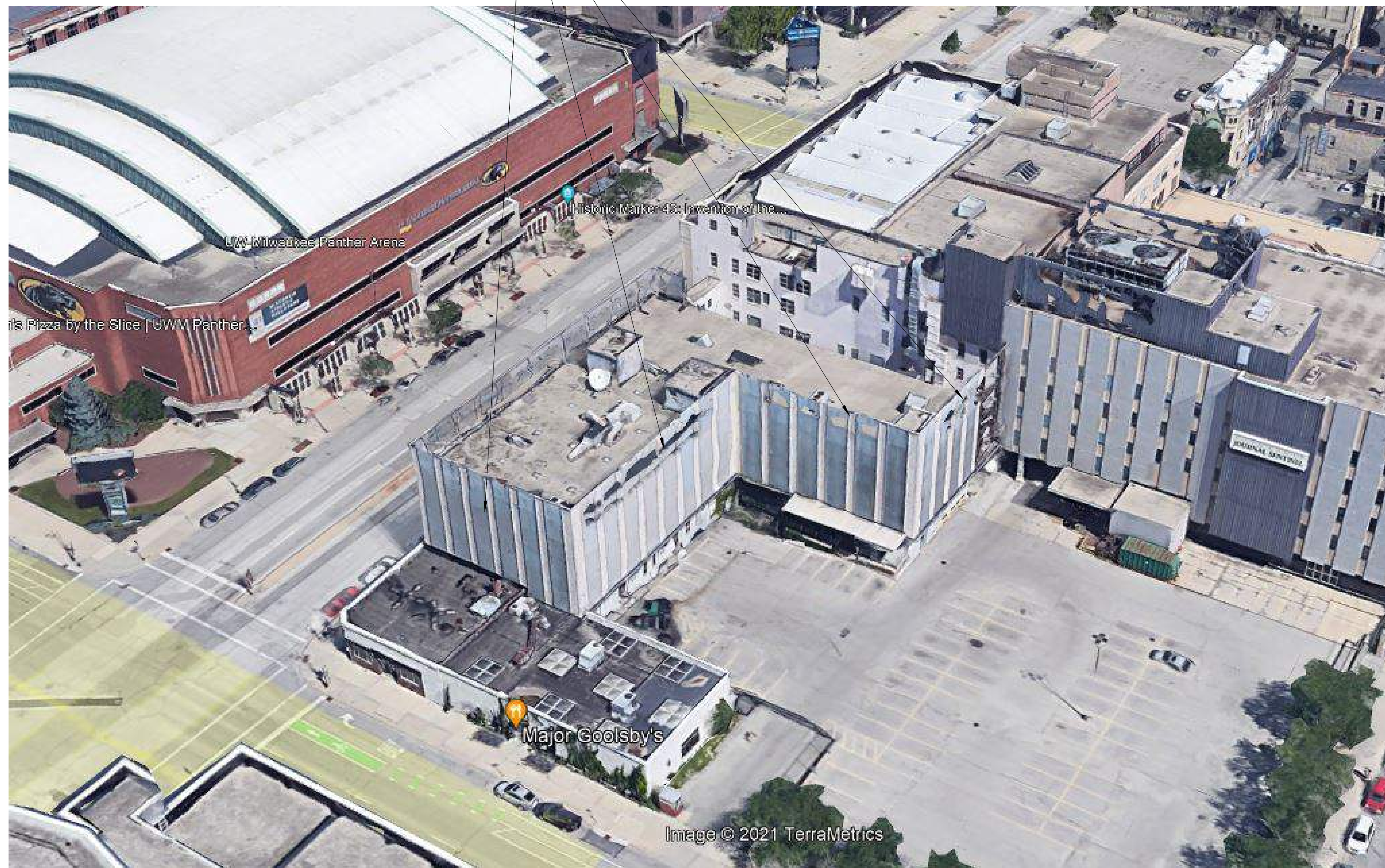
CURRENT SOUTH AERIAL
