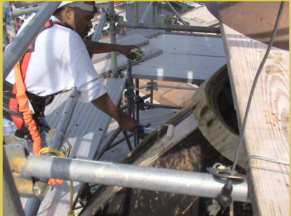
Installation of Wood Battens on the Dome
