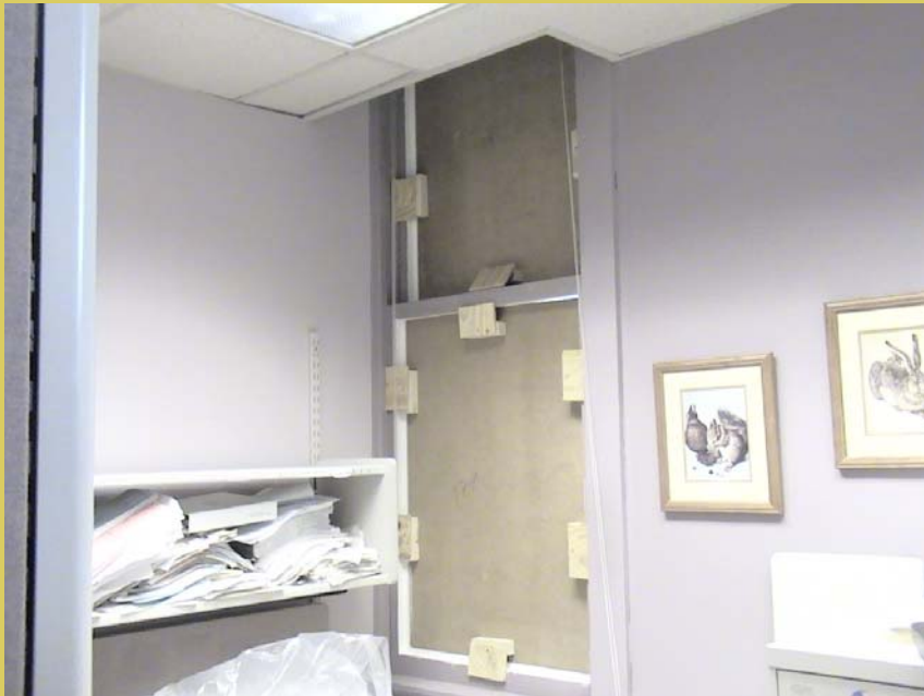
Existing window sashes prepped and primed
