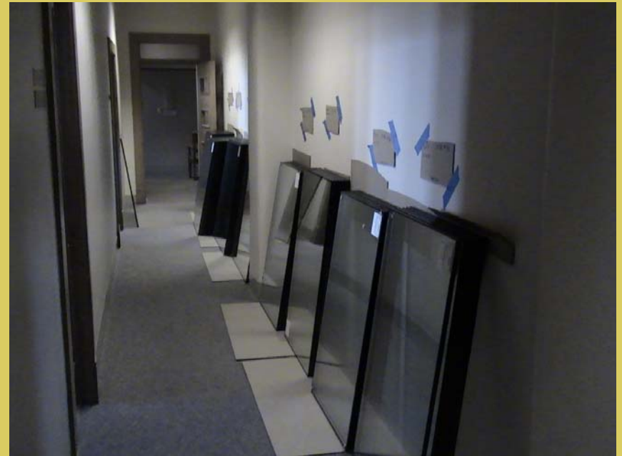
New Insulated Glass Units ready for install
