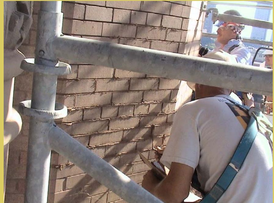
Filling clean mortar joint with new mortar
