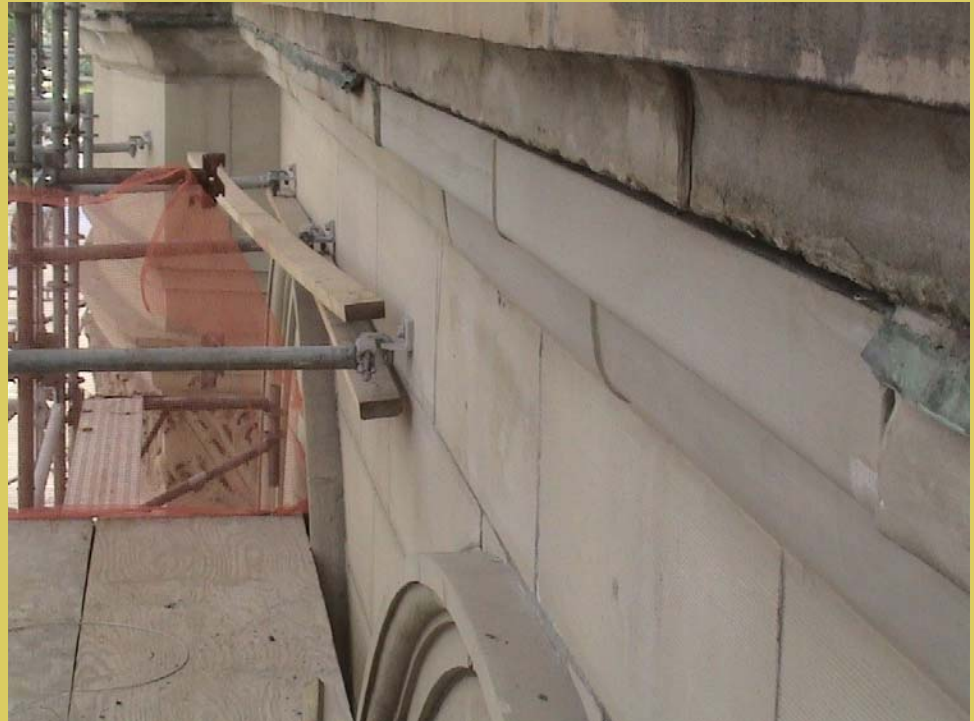
In place Mock-up of Sandstone
