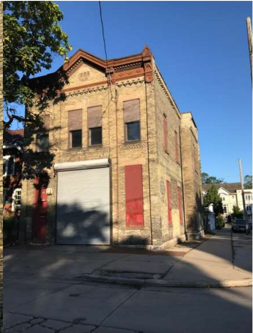
Perspective view of building before construction.
