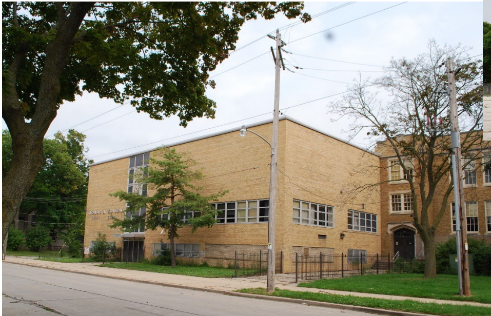
1956 addition, west and south elevations
