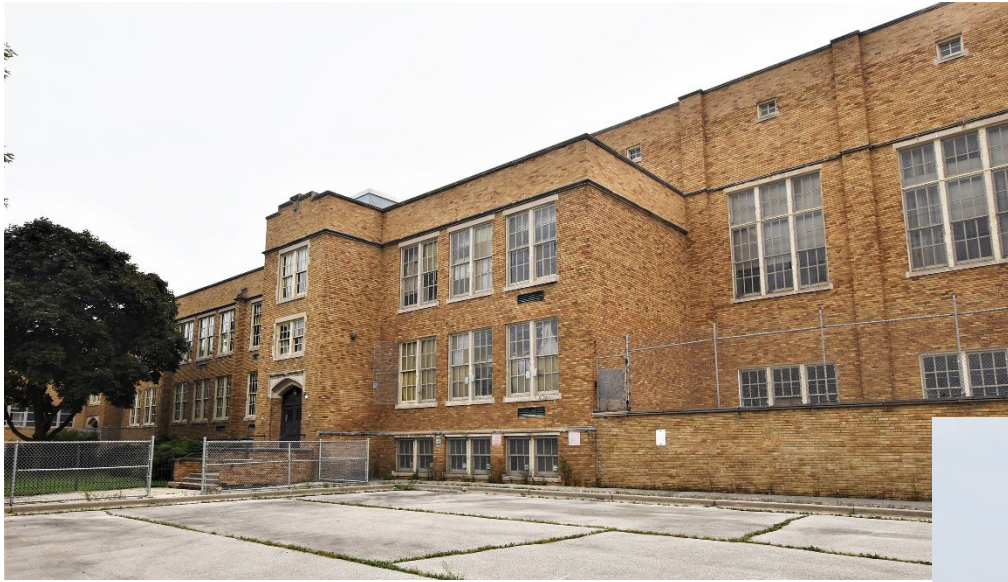
1924 building and 1929 addition, west elevation
