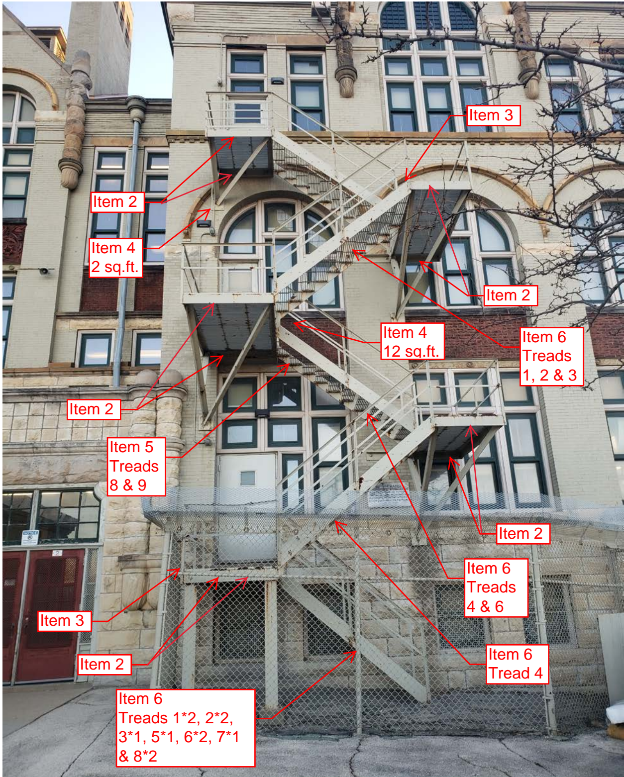
Figure 2 Fire Escape FE#2
