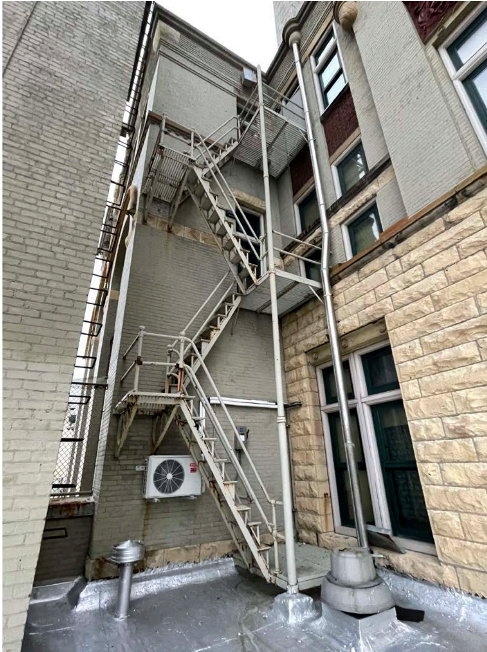
Overall View of Fire Escape #3 (Looking North East)
