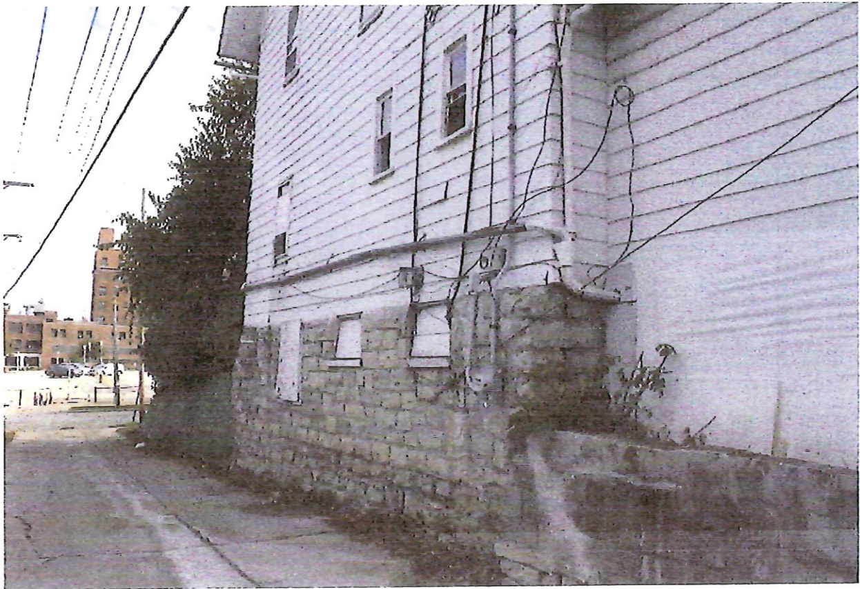
947 N 24 th Foundation – June 2020
