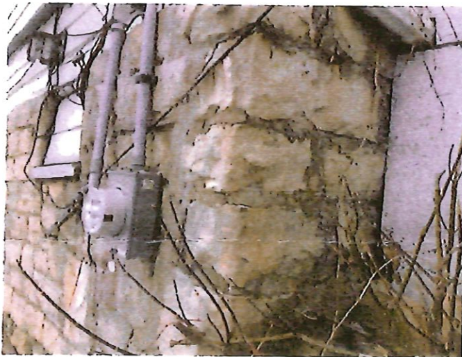
Photo #3 – NW Corner of Basement Wall
