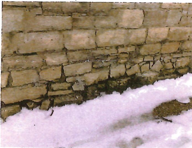
Photo #2 – Base of Basement Wall
