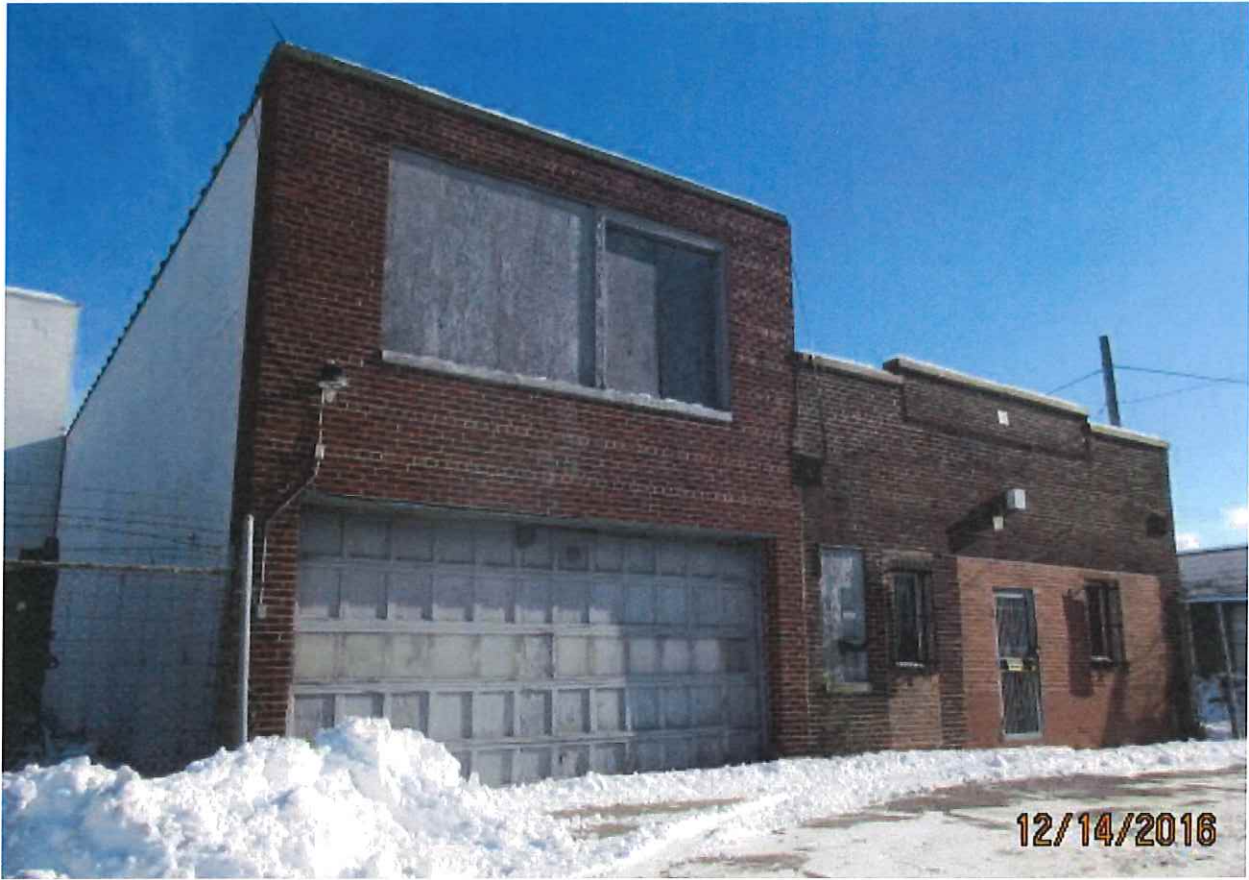
3126 North 31 st Street
