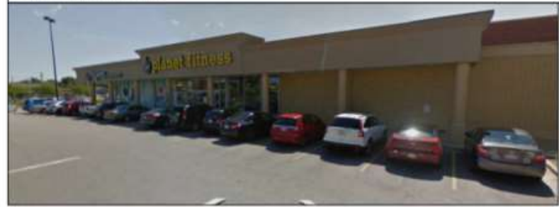
EXISTING NORTH ELEVATION LOOKING WEST
