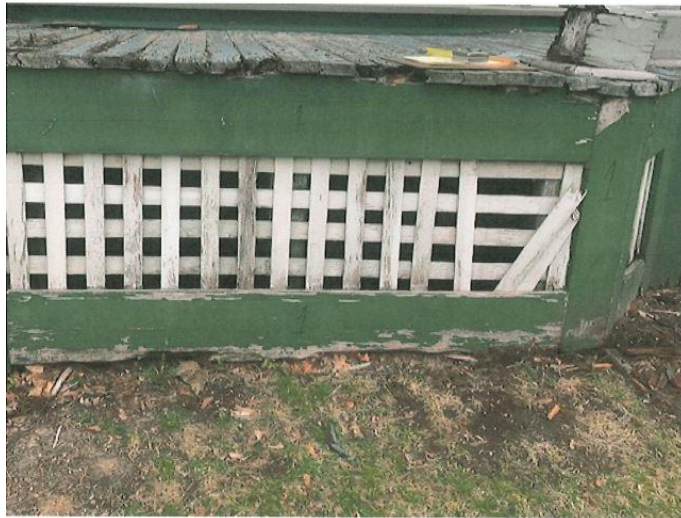
Condition of skirting and decking
