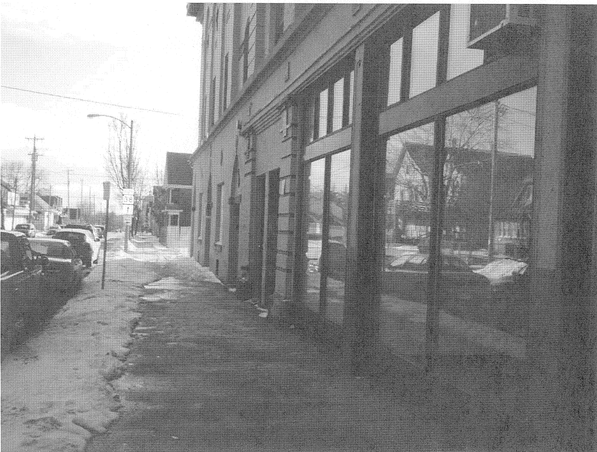
Image 38 - Date: 01-16-2014 – East Elevation (Looking South)
