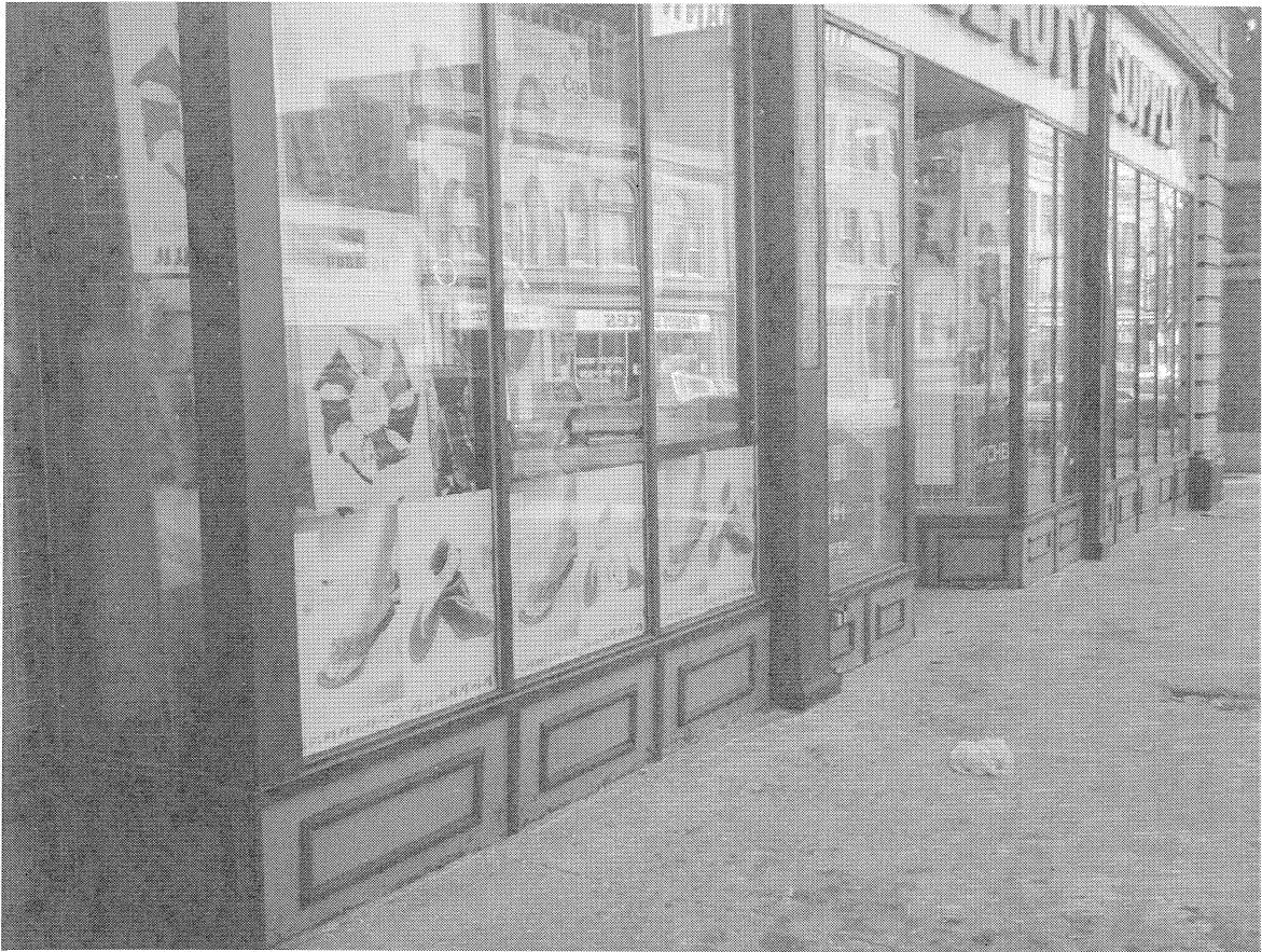
Image 33 - Date: 01-16-2014 – North Elevation (Storefront Base)
