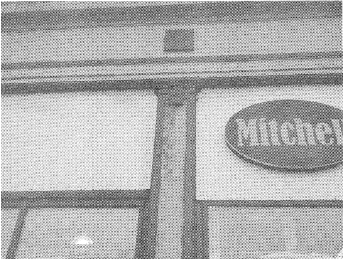
Image 31 - Date: 01-16-2014 – North Elevation (Existing Metal Pilaster with Capital)
