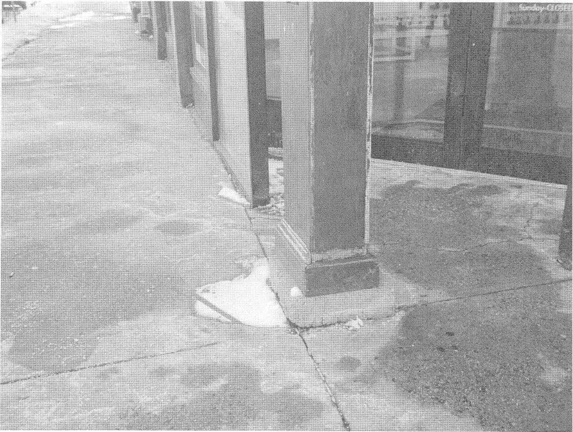
Image 37 - Date: 01-16-2014 – East Elevation (Wood Column)
