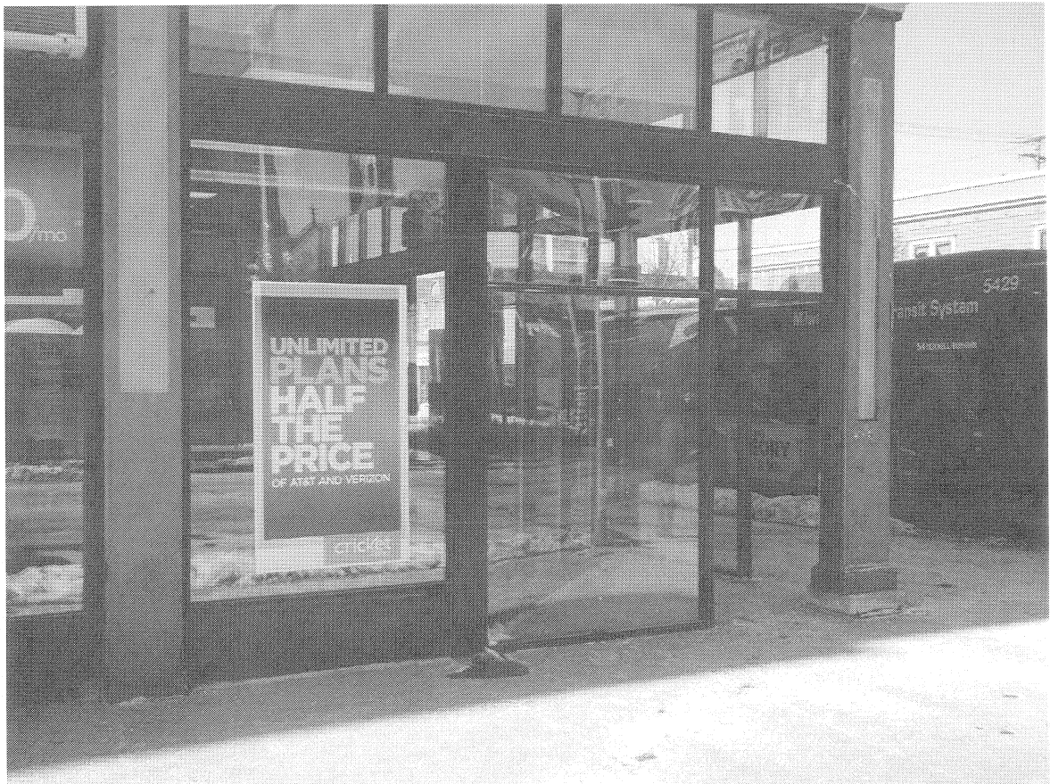
Image 36 - Date: 01-16-2014 – East Elevation (Storefront & Wood Column)
