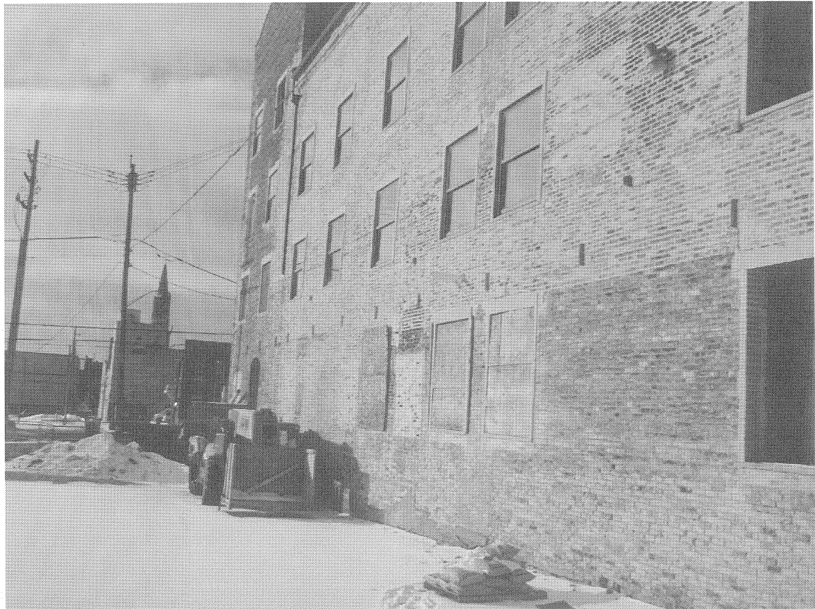
Image 42 - Date: 01-16-2014 – South Elevation (Windows Boarded Up)
