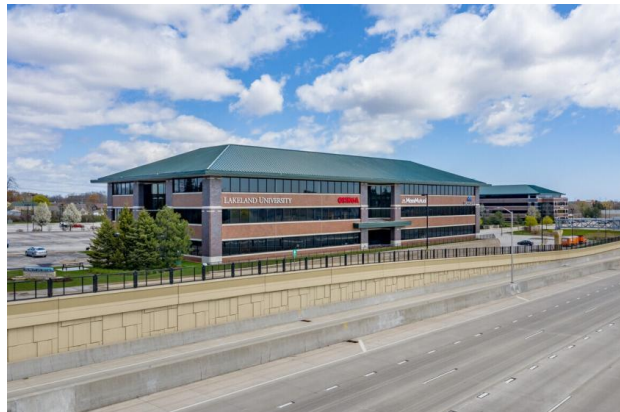
9000 W Chester Street (Phase 4; Ozinga and Lakeland signs have since been removed)
