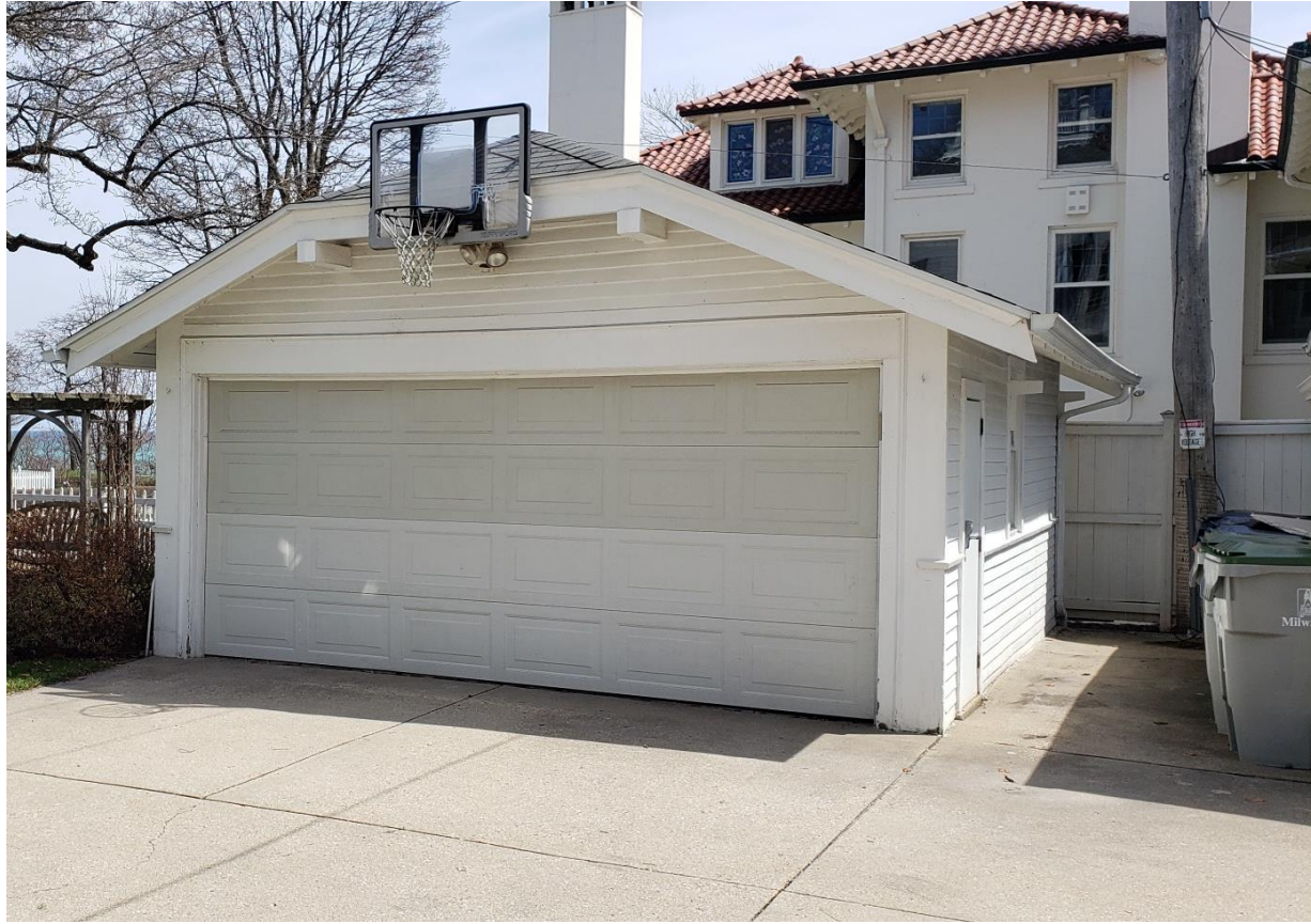
Subject garage near rear lot line.
