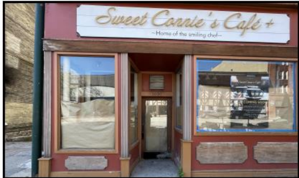
1. STREET LEVEL LOOKING WEST
