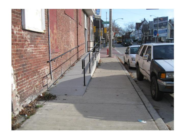
CCF 101302 2301 North Holton Street 12/2/2011 Looking east at ramp structure in north sidewalk area of East North Avenue. There is more than 5 feet of clearance between the ramp and the back of curb.
