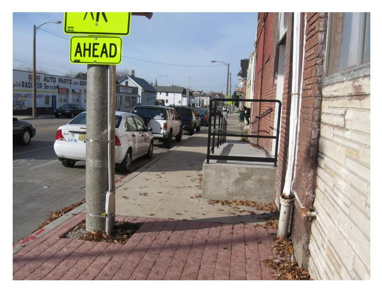
CCF 101302 2301 North Holton Street 12/2/2011 Looking west at ramp structure in north sidewalk area of East North Avenue. There is more than 5 feet of clearance between the ramp and the light pole box out.
