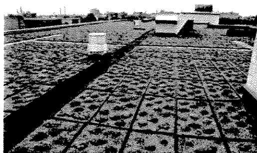
Figure 1: Highland Gardens Green Roof
