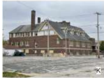
ALLEY VIEW, REAR OF ST. MATTHEW CME CHURCH, 2344 N. 9TH ST
