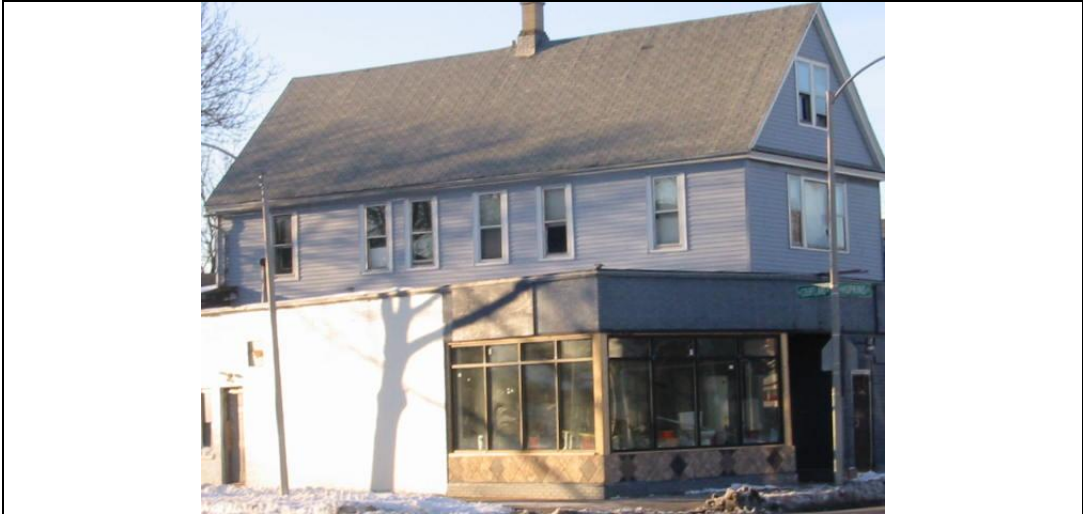
NEW RENOVATED HOME OF BEST CHOICE MECHANICALS AT 4703 NORTH HOPKINS STREET
