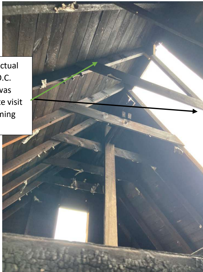
Picture 1: Existing Roof Framing.
