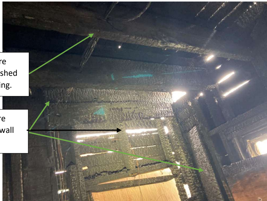
Picture 3: First Floor Southeast Fire Damage.
