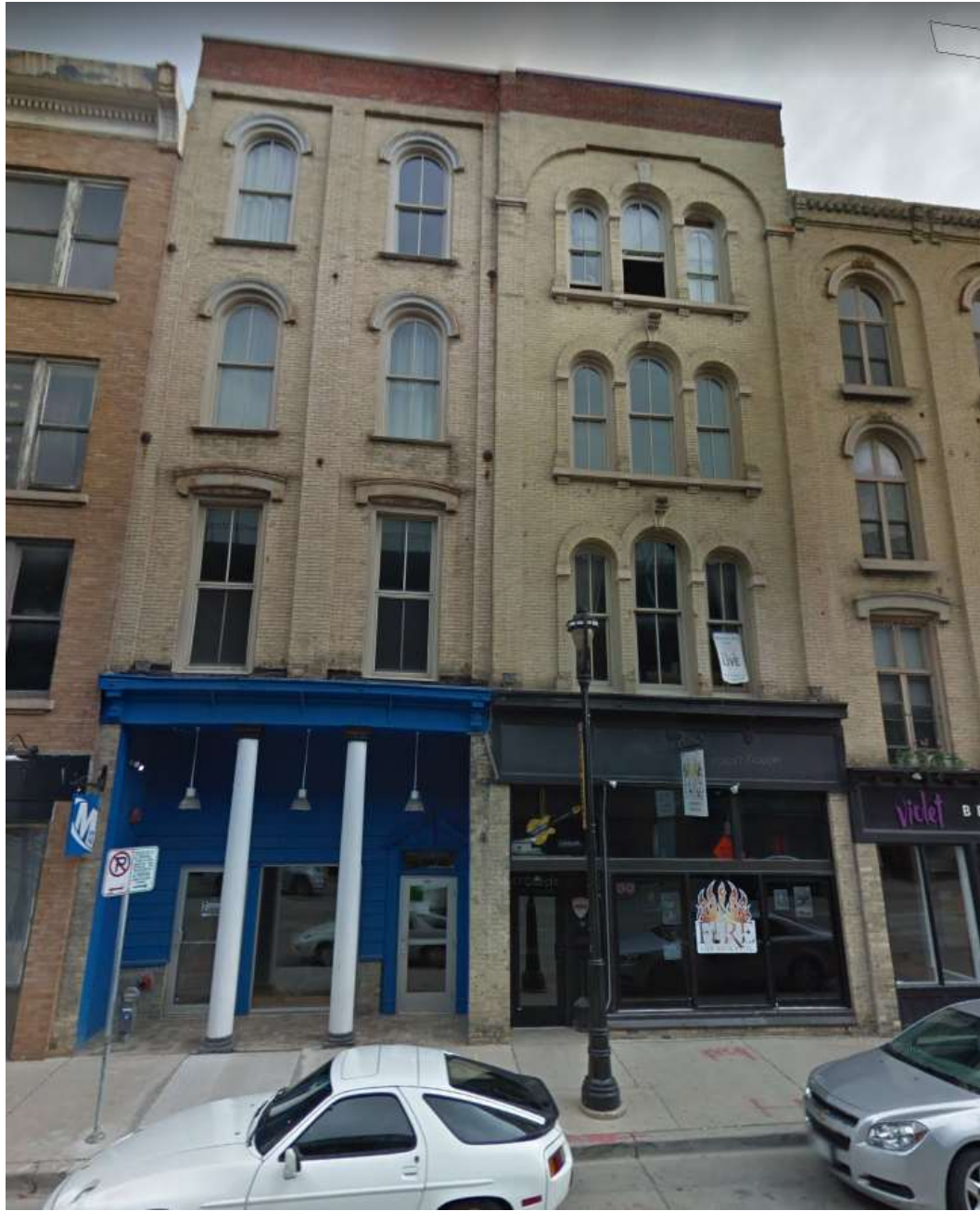
Front of Building
