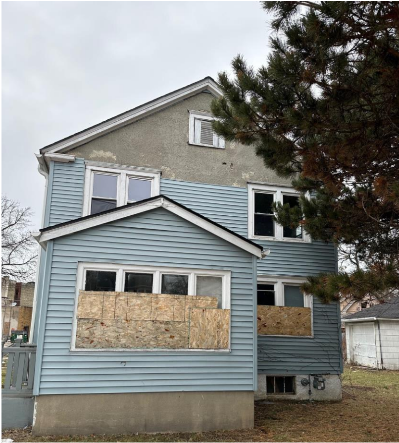
House existing conditions. House to be re-clad with genuine Portland cement stucco.
