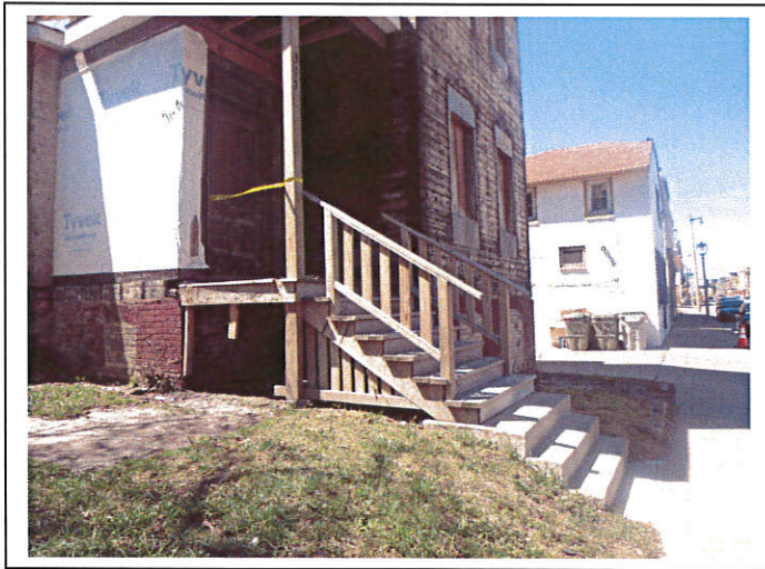
Existing North East Corner Elevation Area where new ADA chair lift will be installed
