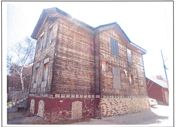
Existing North West Corner Elevation
