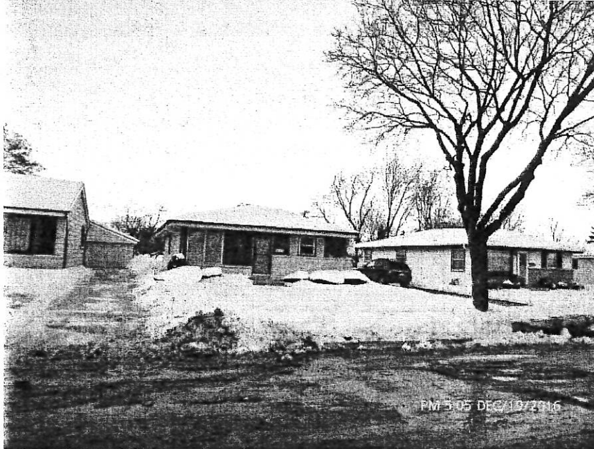
Exterior of home
