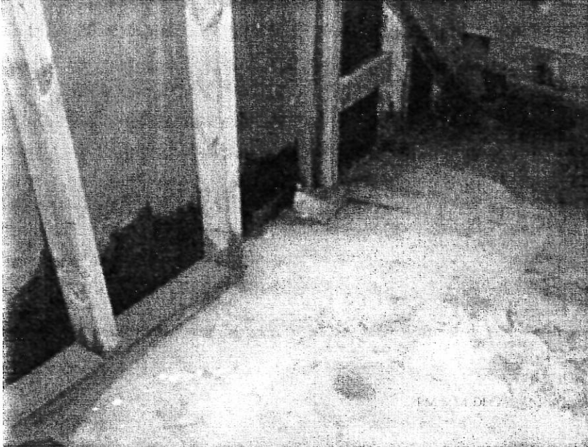
paneling under stairs
