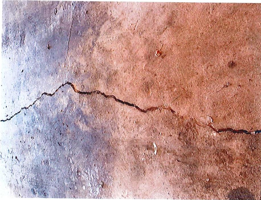
Garage floor cracked. Caused doors not to function.
