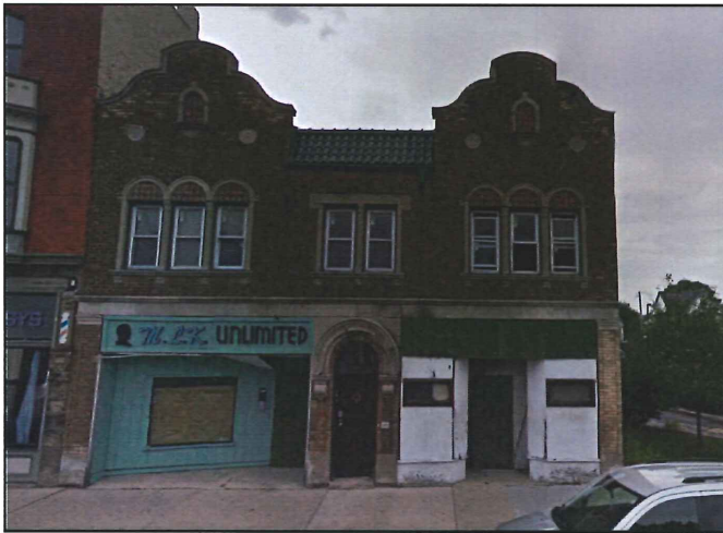
Front view of project site, looking west
