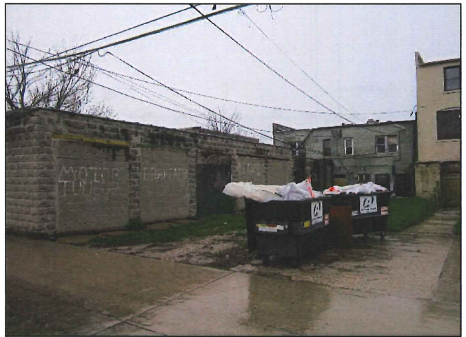
Rear view of project site, looking northeast
