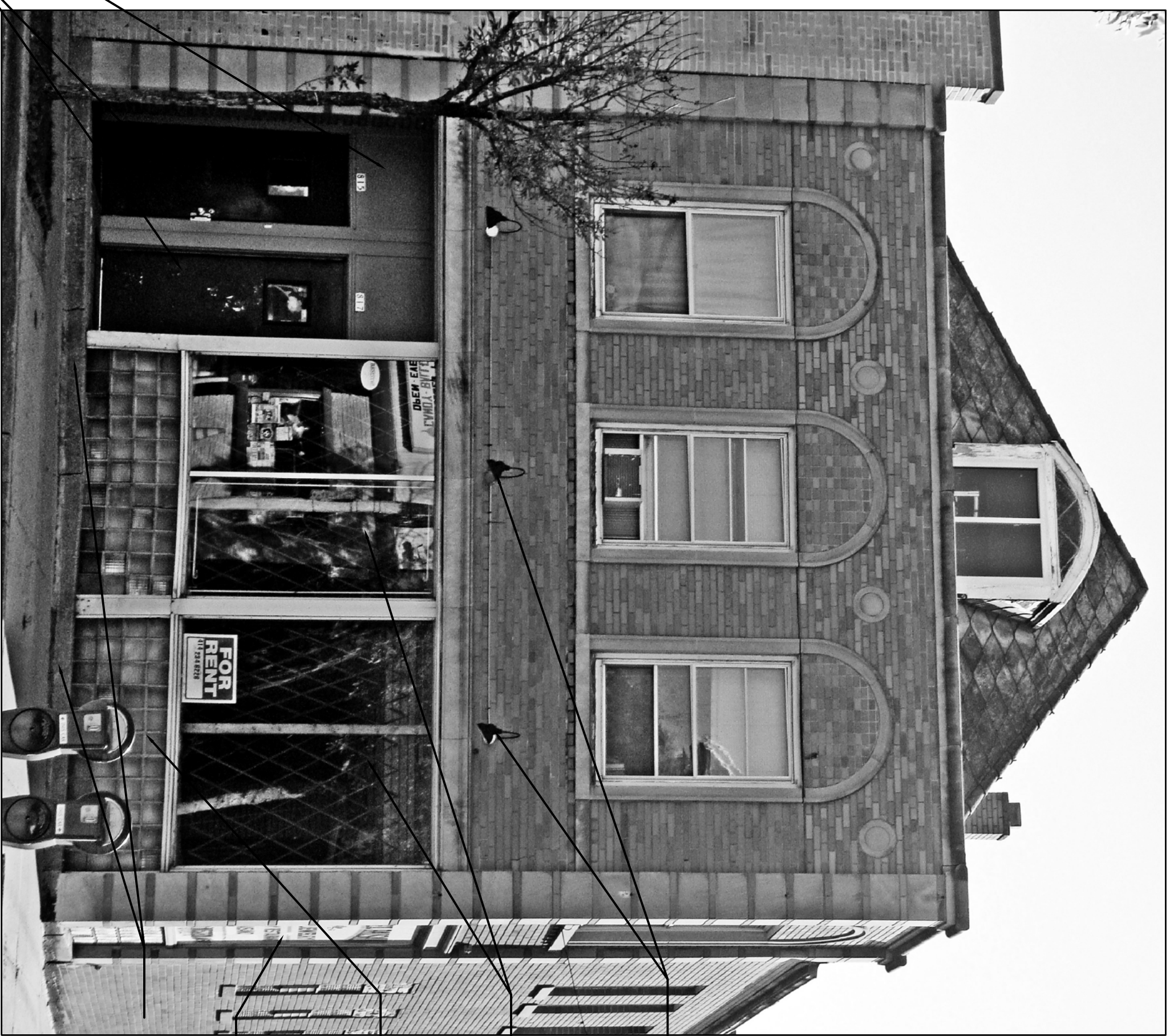
1 REMOVE EXISTING DOORS REMOVE EXISTING TRANSOM PANELS ABOVE BOTH DOORS EXISTING NORTH ELEVATION SCALE: N/A
