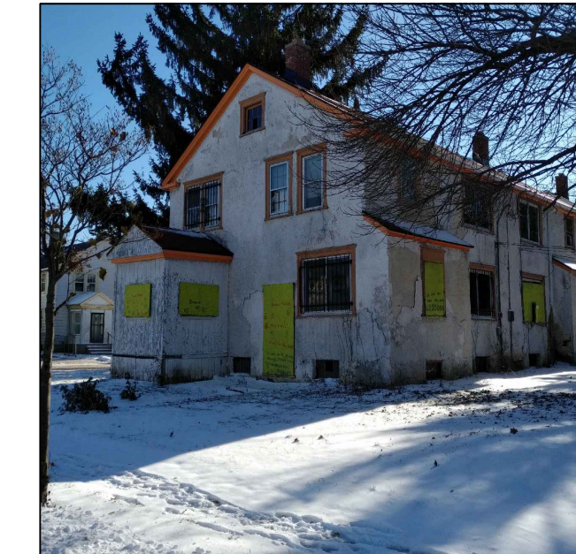
NORTH WEST VIEW
