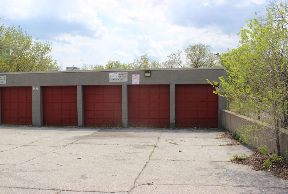
Block A existing structure
