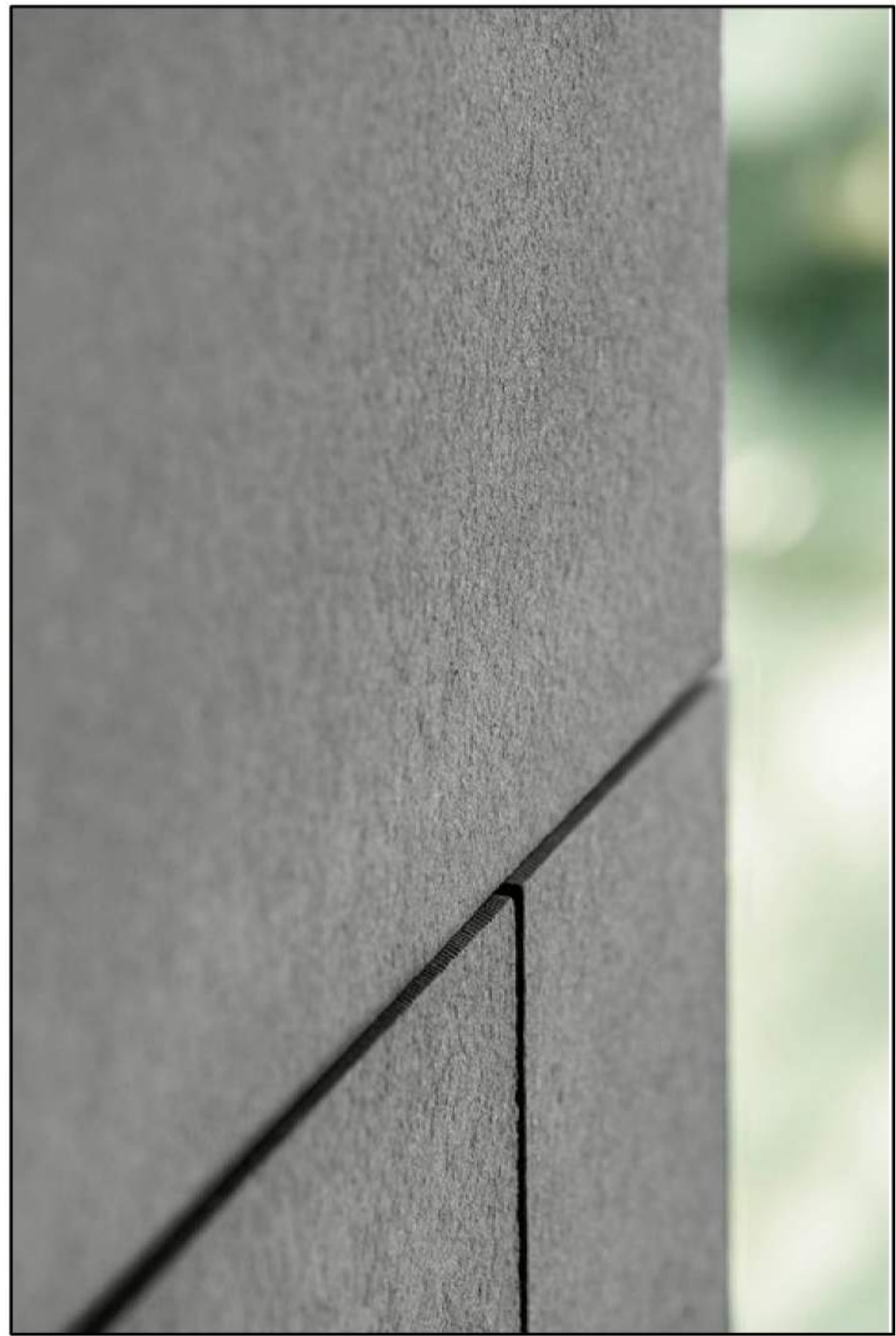
04 FCMT-01 MATERIAL: FIBER-CEMENT WALL PANELS COLOR: CLR-03 SIZE: AS SHOWN FINISH: VERIGATED CONCRETE "WET LOOK" FINISH LOCATION: 2ND THRU 7TH FLOORS
