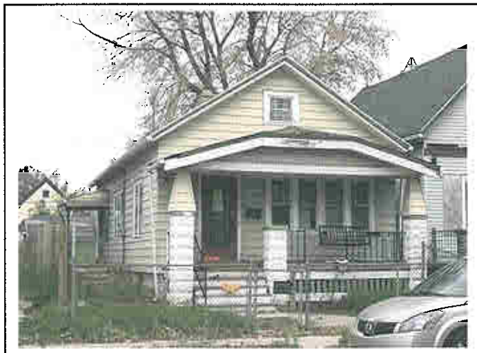
1540 W. Mineral St. – Front View
