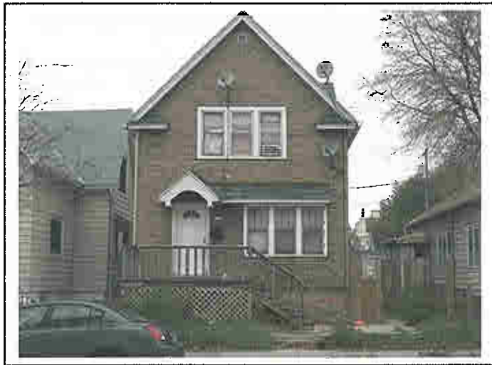
1542 W. Mineral St. – Front View
