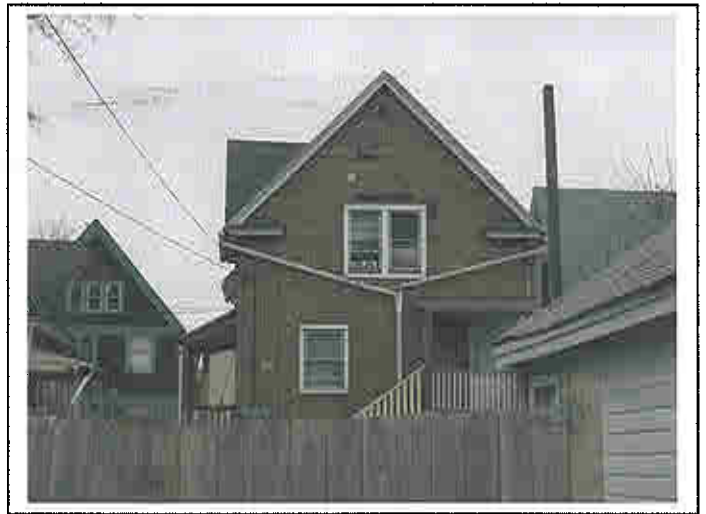
1542 W. Mineral St. – Rear View
