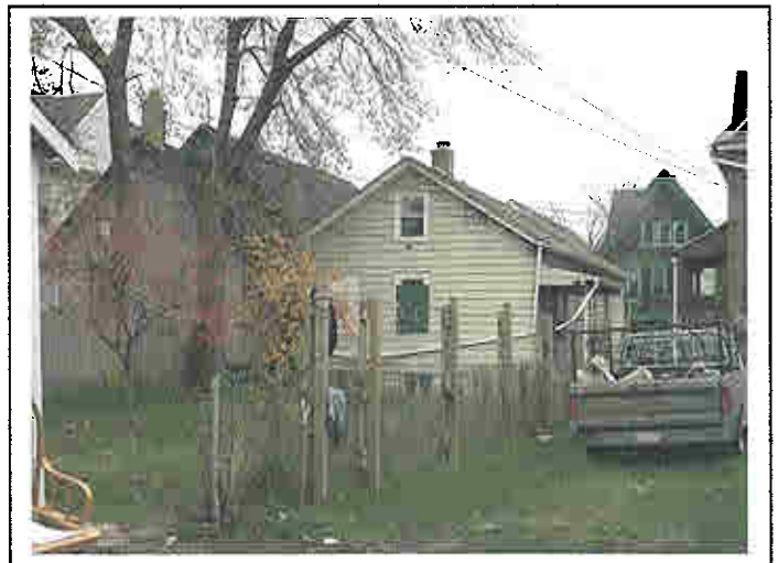
1540 W. Mineral St. – Rear View
