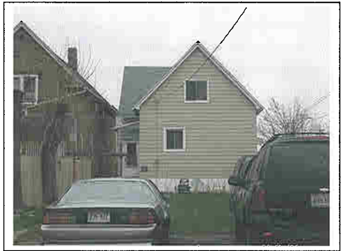
1546 W. Mineral St. – Rear View
