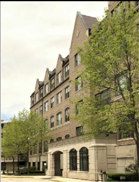
South elevation from alley
