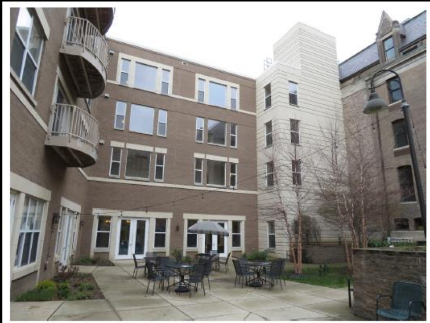
Contemporary Commons Courtyard – location of ramp addition
