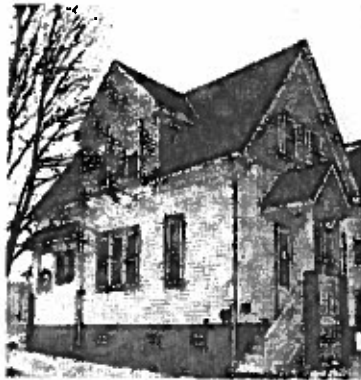
2yr old roof in perfect shape installed by Infinity
