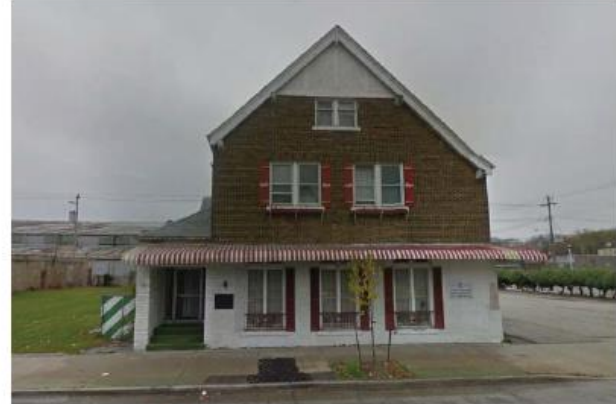
View of 3621 W. Villard Avenue
