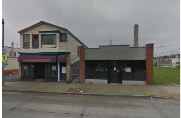
View of 3605-3611 W. Villard Avenue
