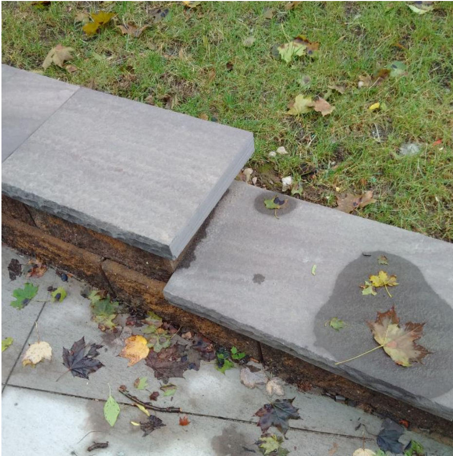
Images of the new retaining wall cap (red Chinese sandstone installed as directed by HPC staff)
