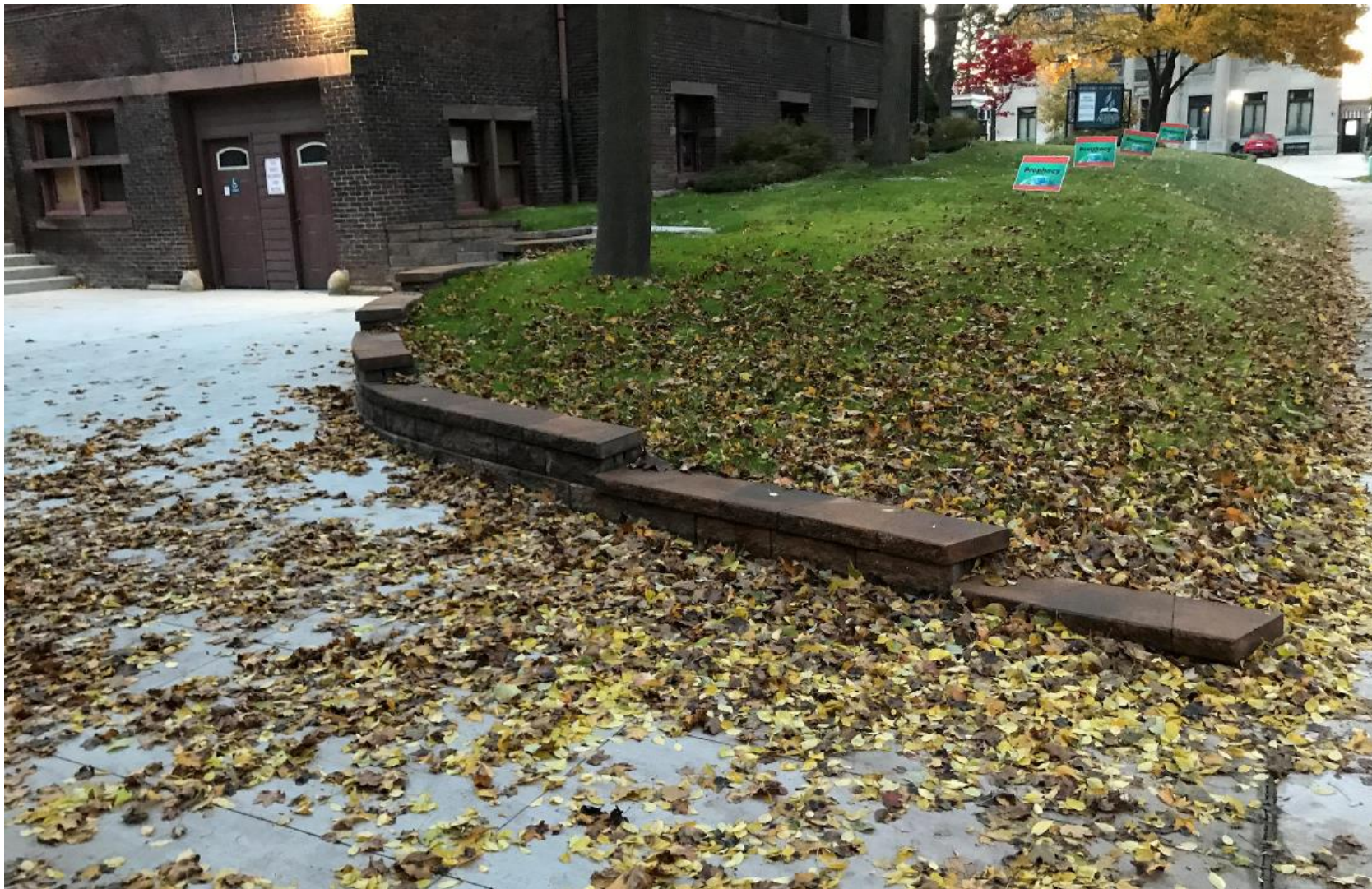
Previous condition (retaining wall capped with concrete)
