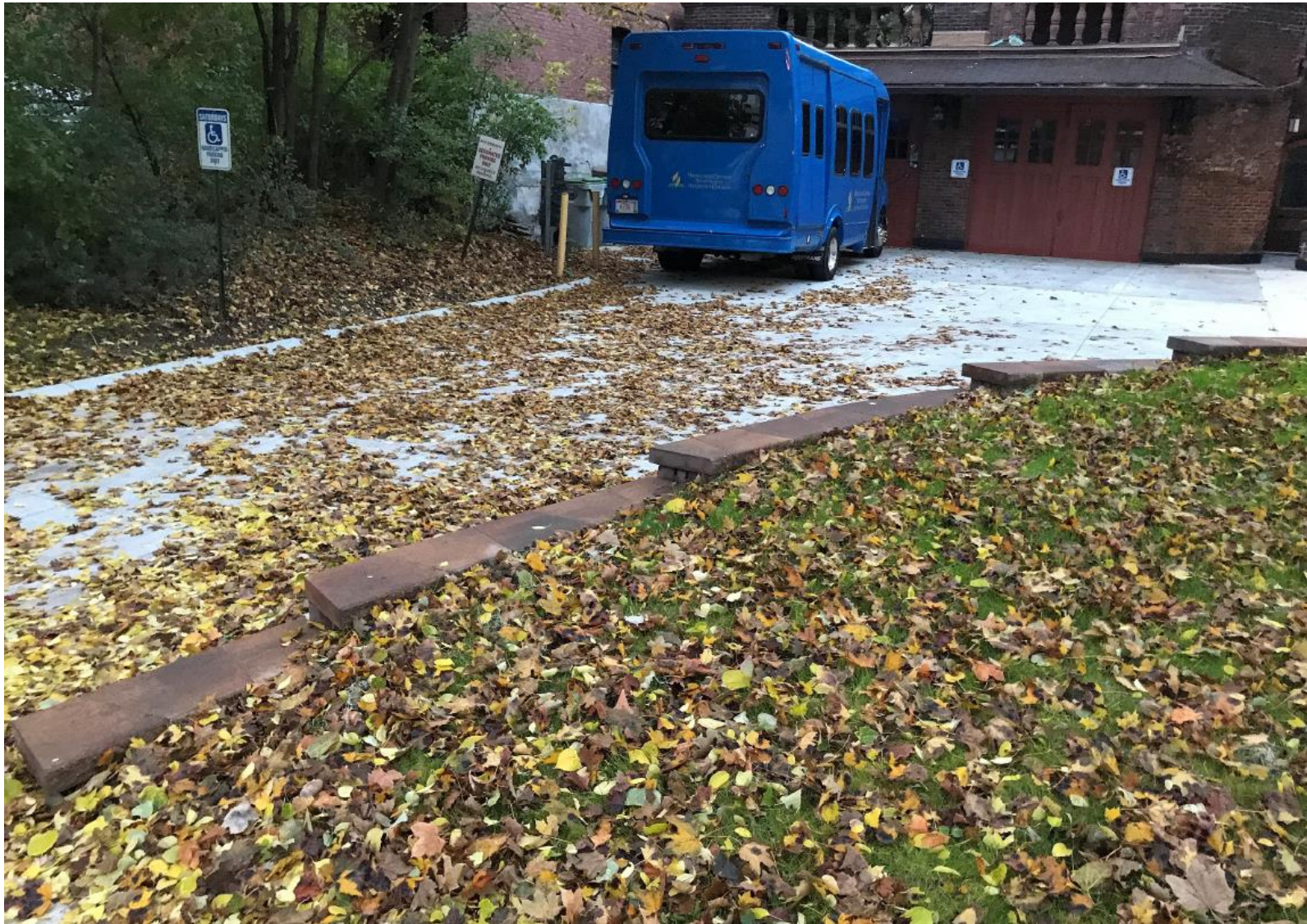
Alternate view of previously existing concrete caps on retaining wall
