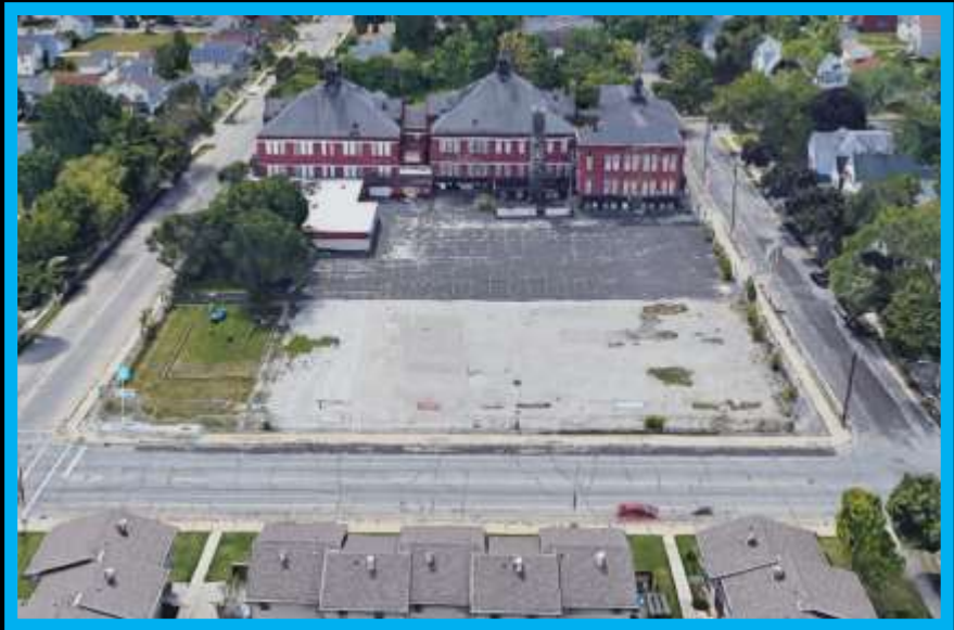
Aerial view looking south
