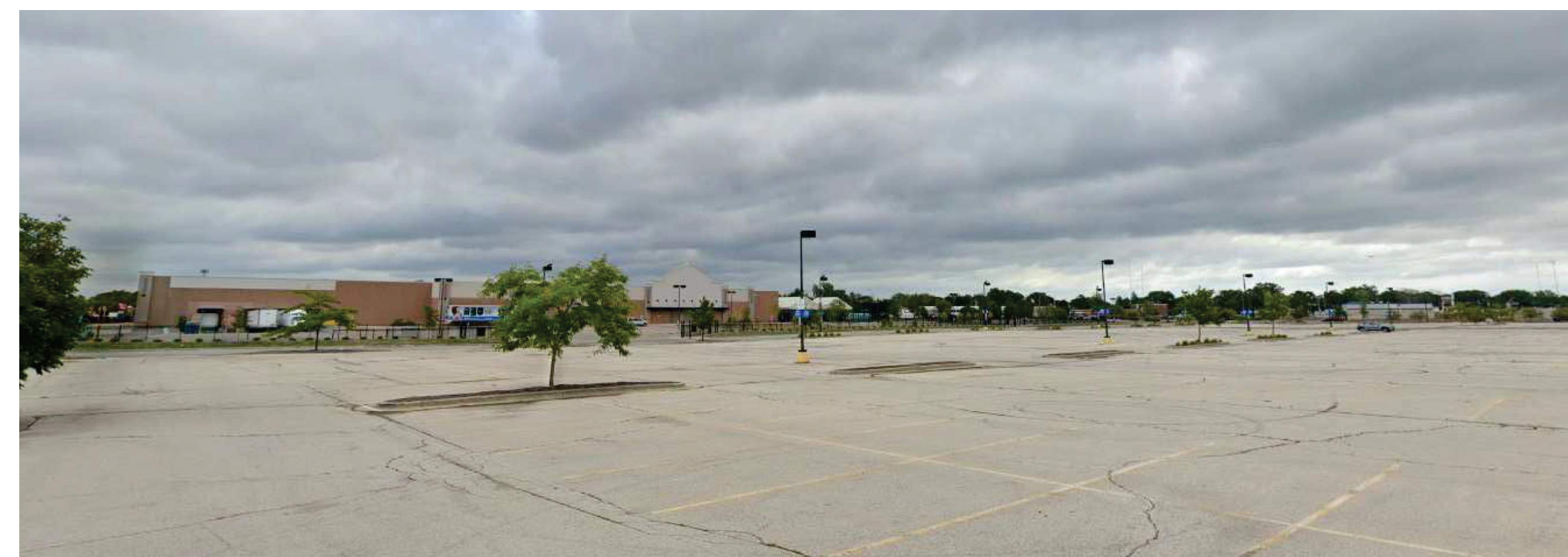
LOCATED AT NORTHEAST CORNER OF NORTH PARKING LOT LOOKING SOUTH TOWARD EXISTING BUILDING
