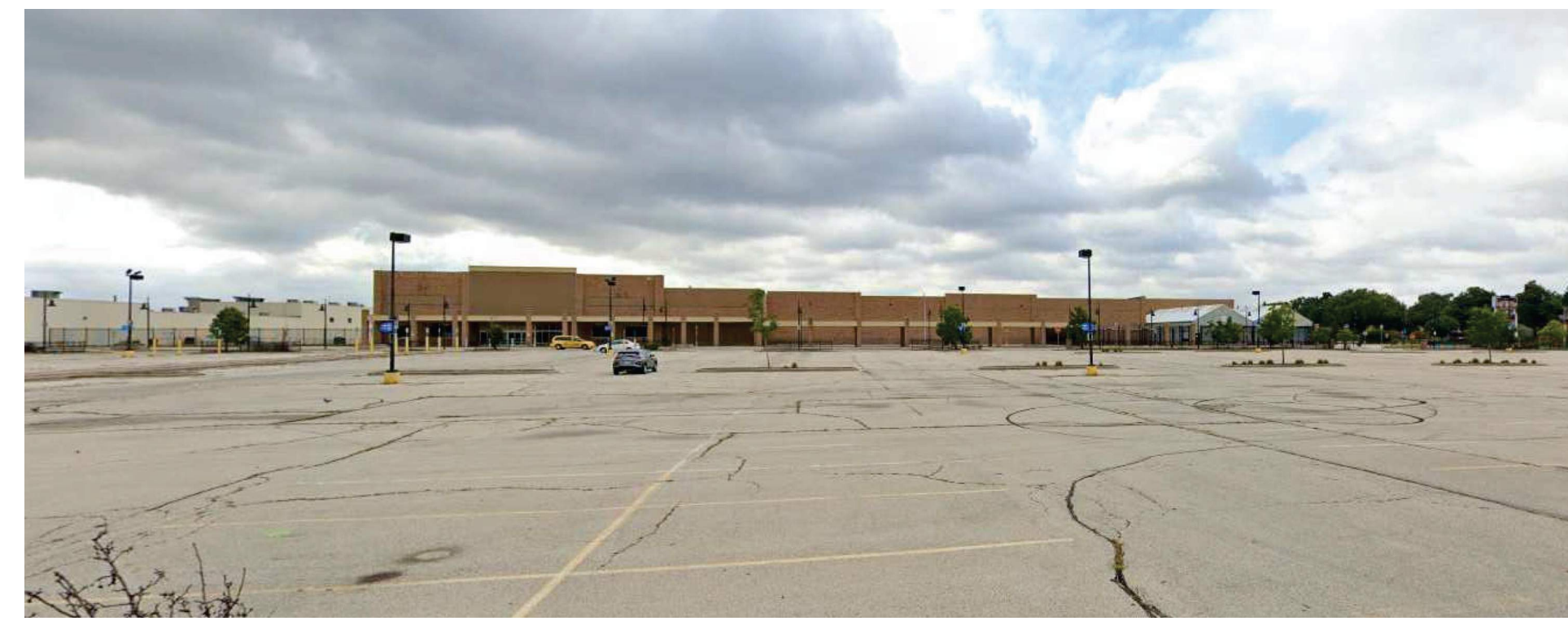
NORTH FACE OF EXISTING BUILDING
