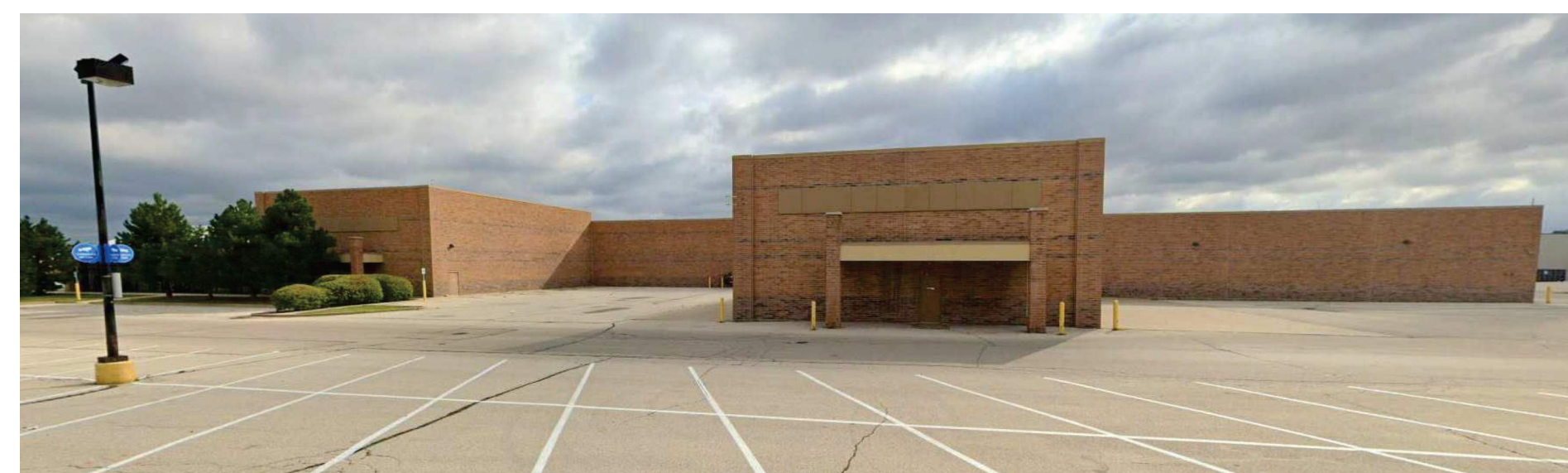
WEST SIDE OF EXISTING BUILDING
