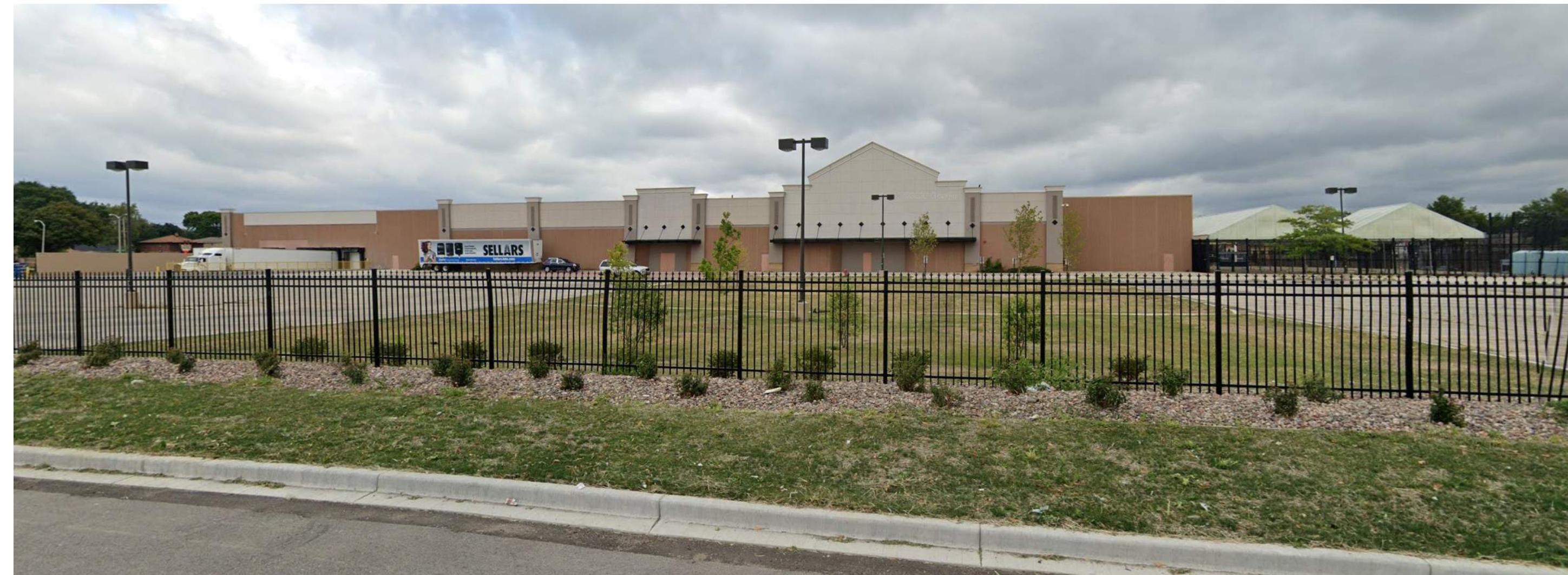
EXISTING MIDTOWN CENTER - SELLARS ABSORBENT MATERIALS PLANT #3, LOOKING NORTH (PHOTO FROM GOOGLE MAPS, SEPTEMBER 2019)
