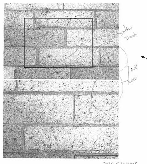
Sample of new mortar that will match the old in terms of joint color, texture, hardness, joint width and joint finsh.
