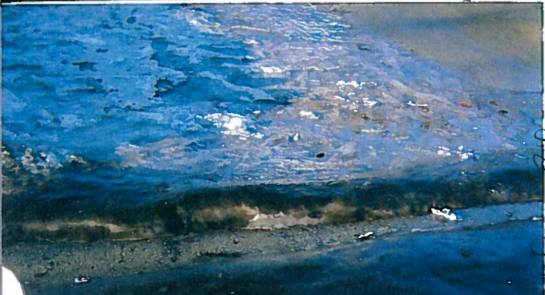
Water draining into the street in front of my property and beyond (going north)
