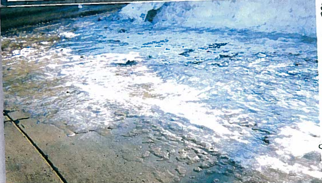
Ice buildup and mud debris settled on lot, (stalls 5 & 6)
