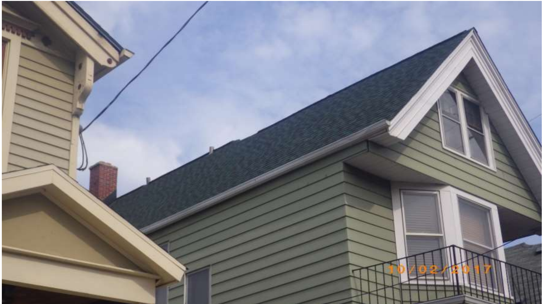
Roof and chimney after project completion. Note ridge venting.
