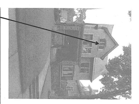
Restore third floor front gable windows using structural wood epoxies (auto body filler must NOT be used). Windows must be painted upon completion
