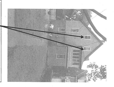
Rear windows in gable will be replaced with new, matching, all-wood windows. See attached shop drawings. New glass sizes must match the originals and the designs of the new window must match the originals.
