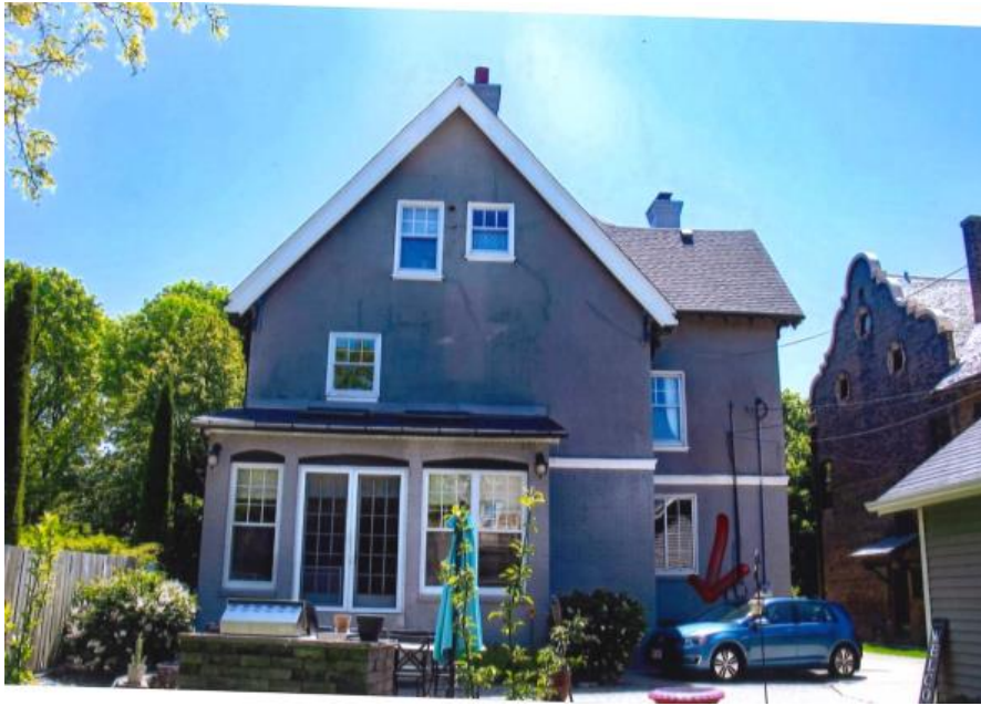
Location of AC unit to be replaced on rear facade
