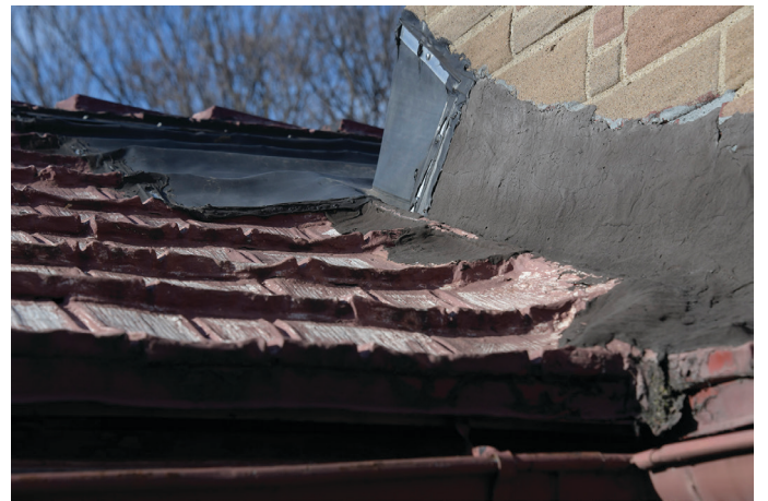
Model C3 Leaking roof - 5 layers, including the original layer of wood shingles (circa 2022)
