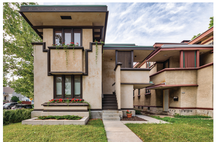
Two Family, "Flat C" Before Restoration
