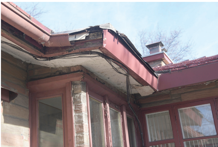
Model C3 Deteriorated roof overhang, gutters, and trim (circa 2022)
