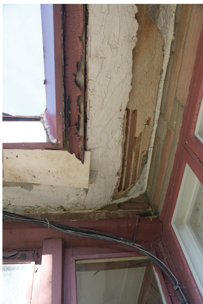
Model C3 Deteriorated roof overhang, gutters, and trim (circa 2022)
