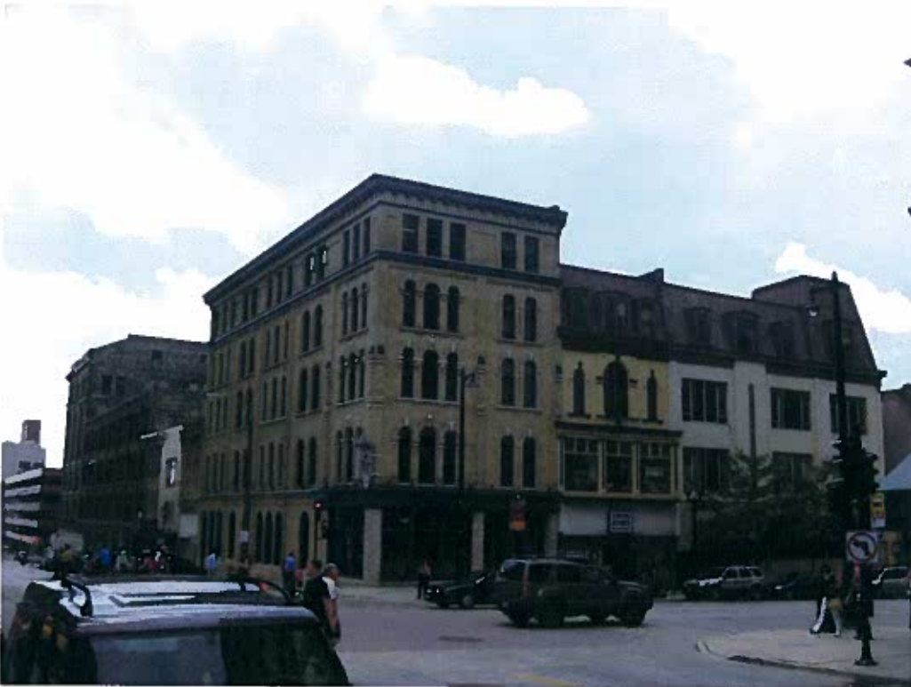
Photo 4: Corner of East Wisconsin Avenue and North Milwaukee Street
